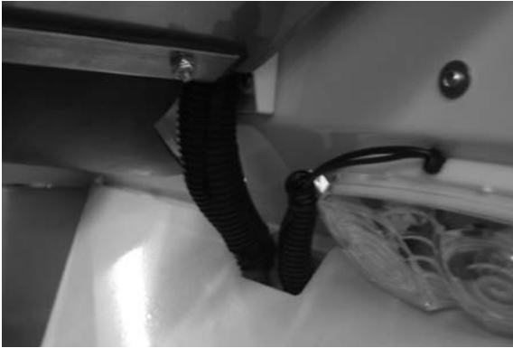
Figure C-8: Cables coming down from top to the base of the HCGG
