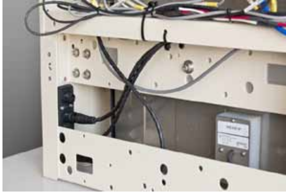
Figure D-4: BDS CAN cable installed
