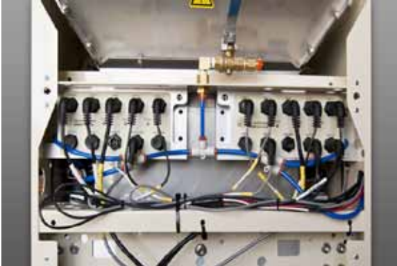
Figure D-3: Cables routed to modules
